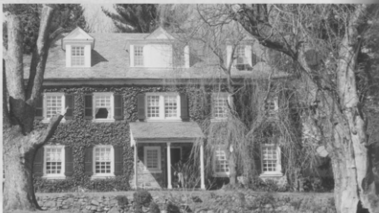
Lot 29. Isaac Jones's house, west side, 1968. Lot 31. Simeon Matlack's house c.1910. Lot 33. Adam Siter's house (left hand portion), 1975.
