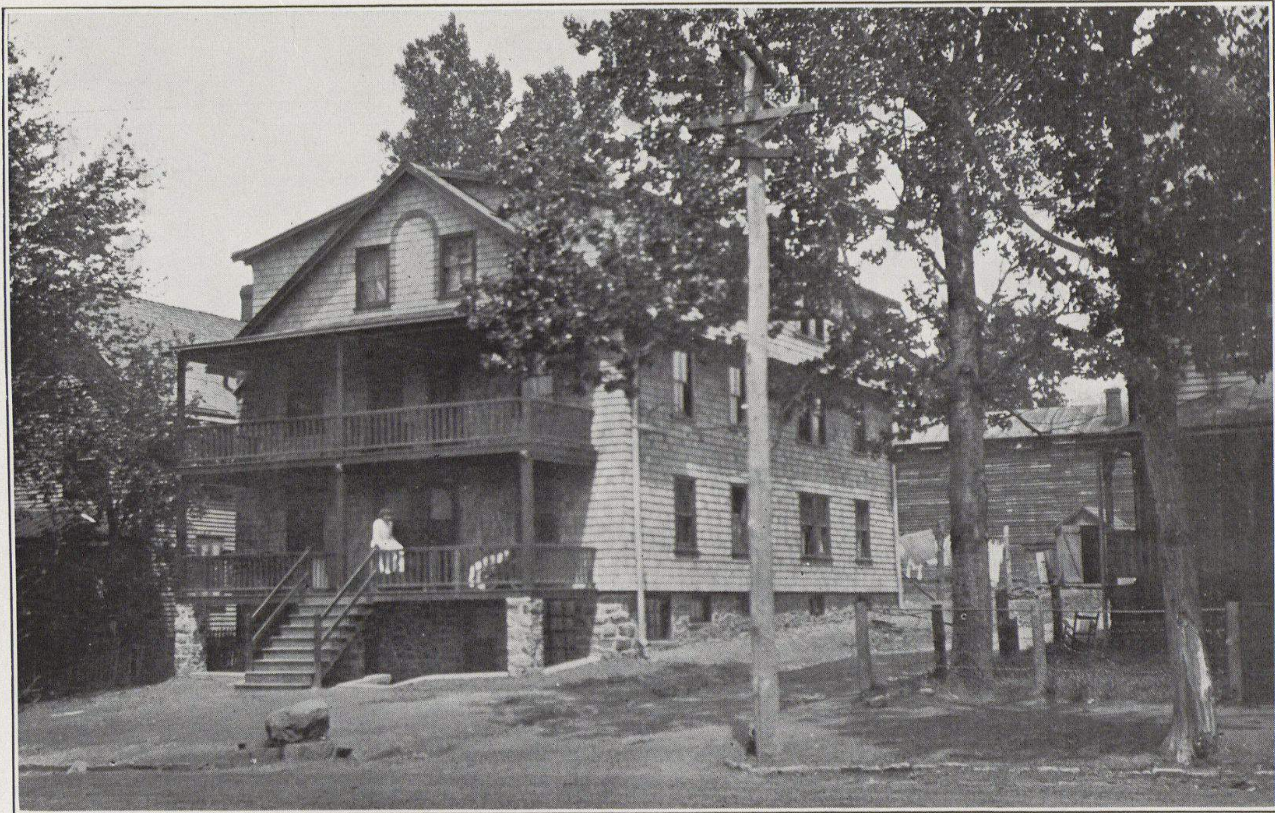
A WAYNE TENEMENT—3 STORIES HIGH—4 FAMILIES ON EACH FLOOR. NO FIRE ESCAPE. THIS BUILDING COULD NOT BE BUILT IN A CITY, BUT THERE ARE NO BUILDING REGULATIONS FOR THE SUBURBAN AREAS.
