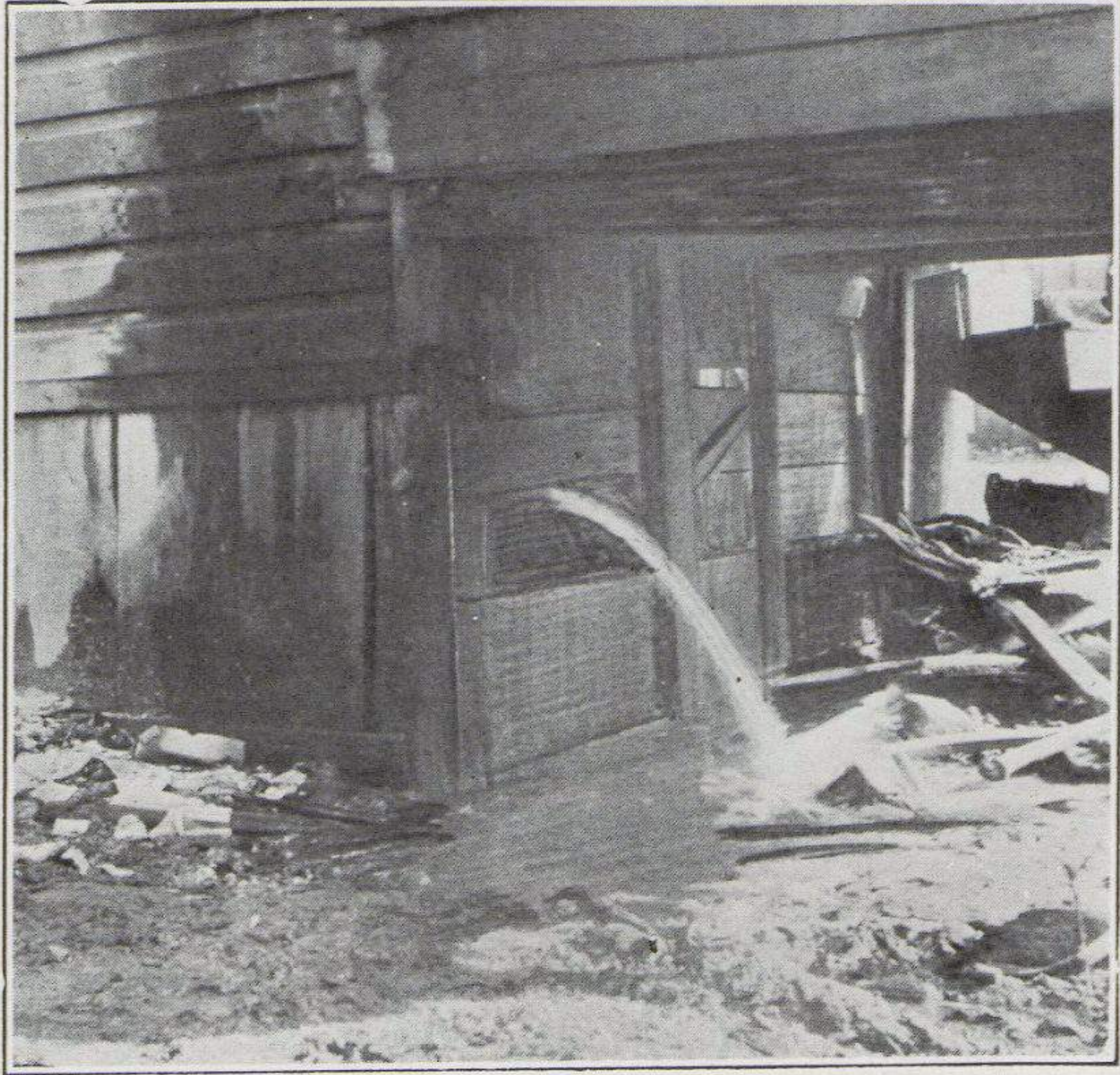
LANCASTER PIKE. House Drain Discharging. Water Flows Beneath House and Causes Stagnant Pool.
