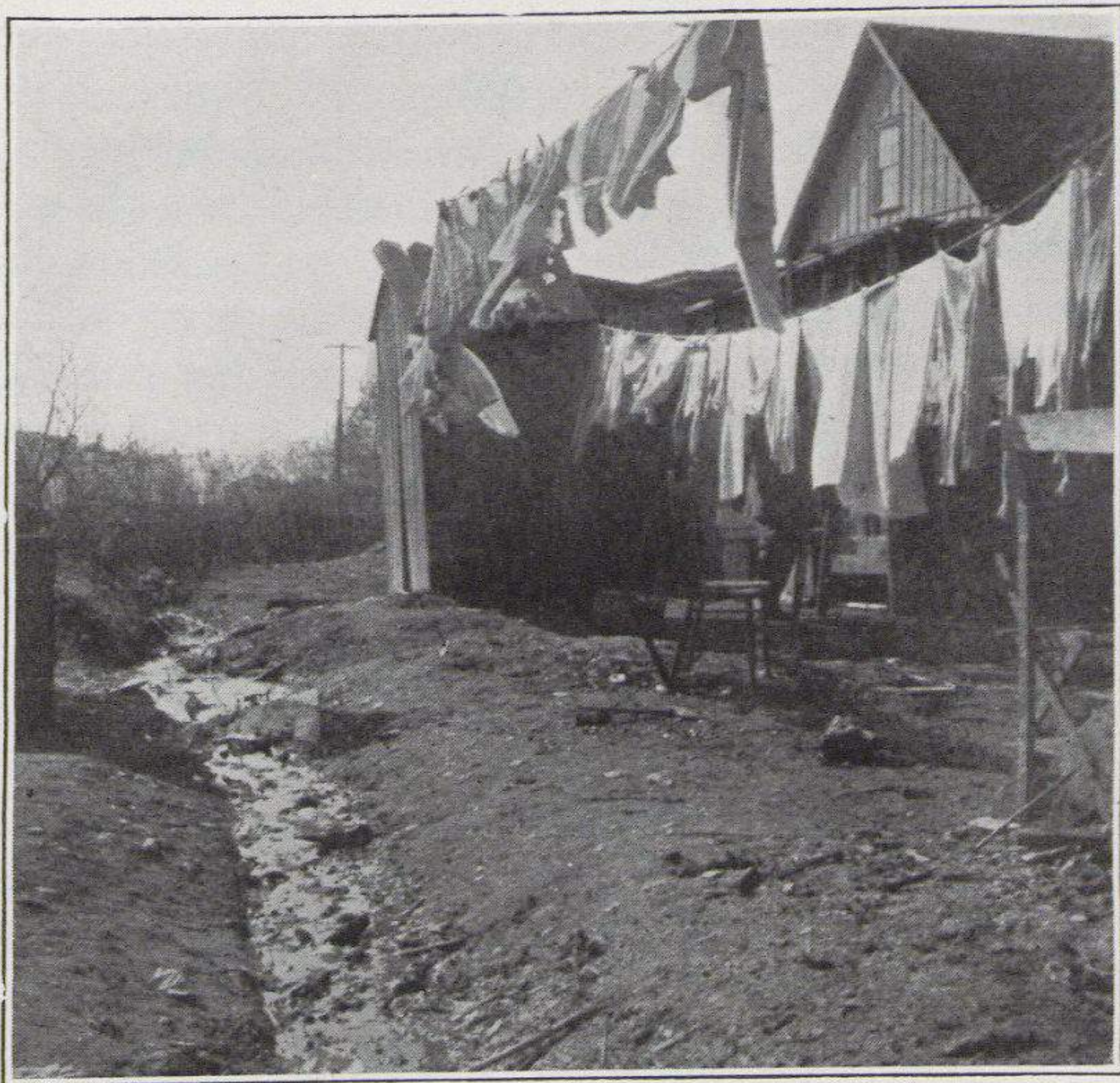
HOUSE SEWAGE DRAIN. Rear of a Row of Shacks on Lancaster Pike.
