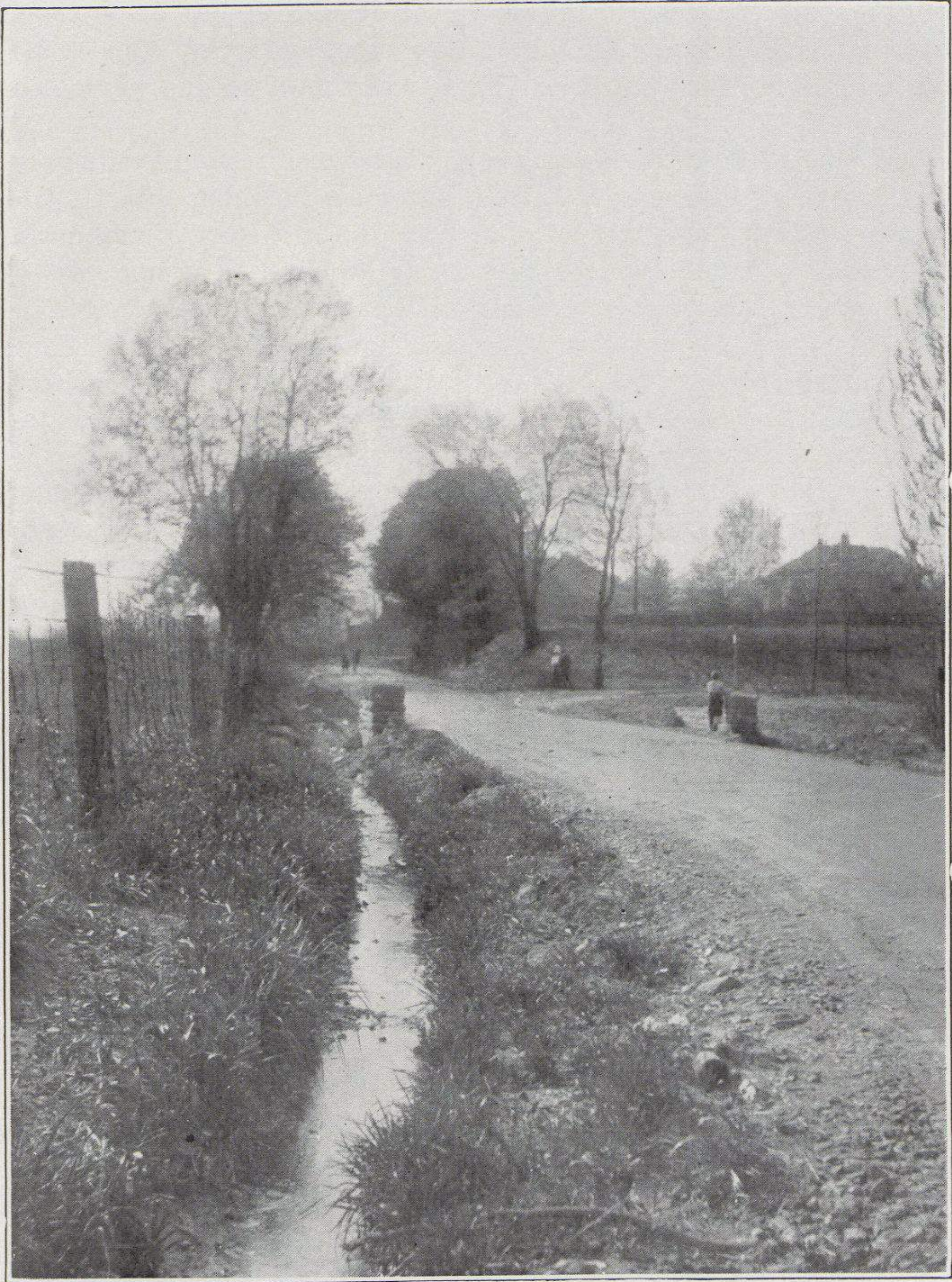
Haverford Road. Surface Drainage from the Surrounding Streets and Houses. A Breeding Place for Mosquitoes. Gutter Very Foul and Filthy with House Sewage.
